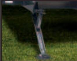
Jacks with sand pad
